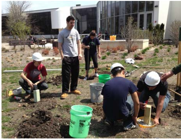
Figure 1.3: The photo below illustrates the students' design solution of creating removable foundations in five gallon buckets.
