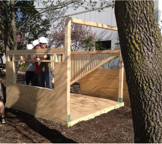
Figure 1.8: The photo below illustrates students working together to frame the walls and roof for the pavilion.
