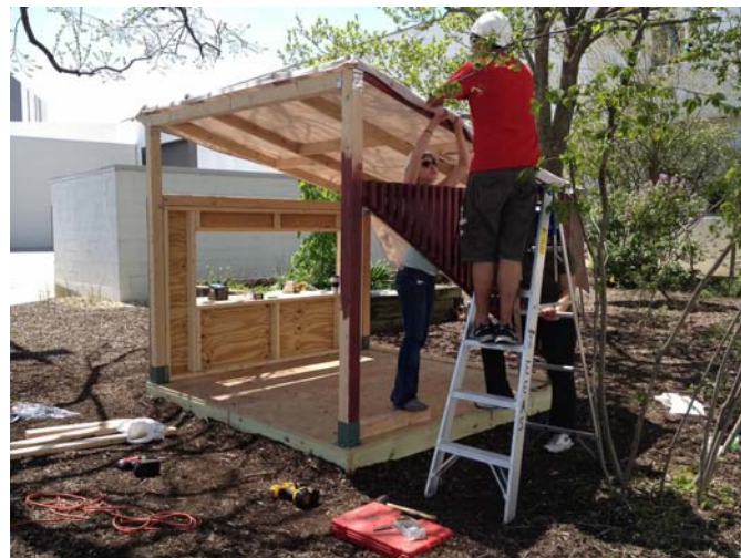
Figure 1.10: The final days of the pavilion construction project.
